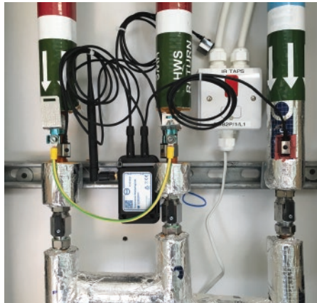
The battery-powered units connect quickly and easily to the water pipe, TMV, or outlet, using small clamps.
